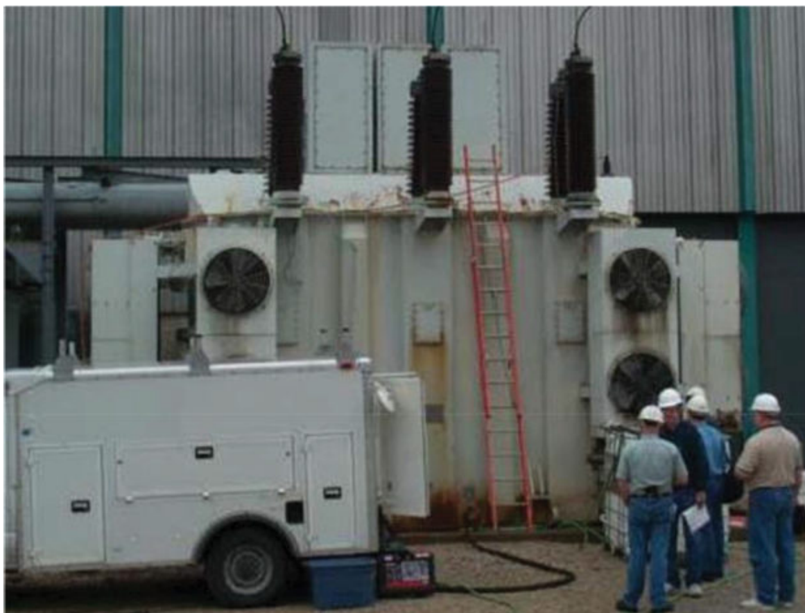
Fig. 8: Generator step-up transformer, rated at 200 MVA and 161 kV, manufactured in 1966 and filled with mineral oil, was retro-filled in 2004 with natural ester fluid.
