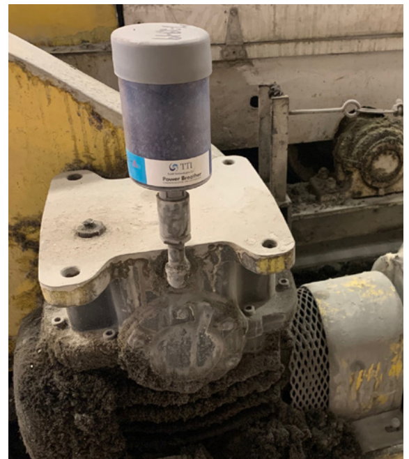
Figure 6. TTI Power Breather Installed
