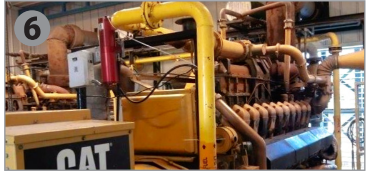
6. This CAT 3520 landfill generator is equipped with a single HI4 Conserver™ Oil Purification Unit.
