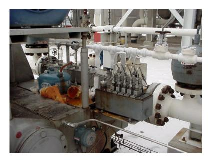
Cylinder No. 2 - Packing Leak
